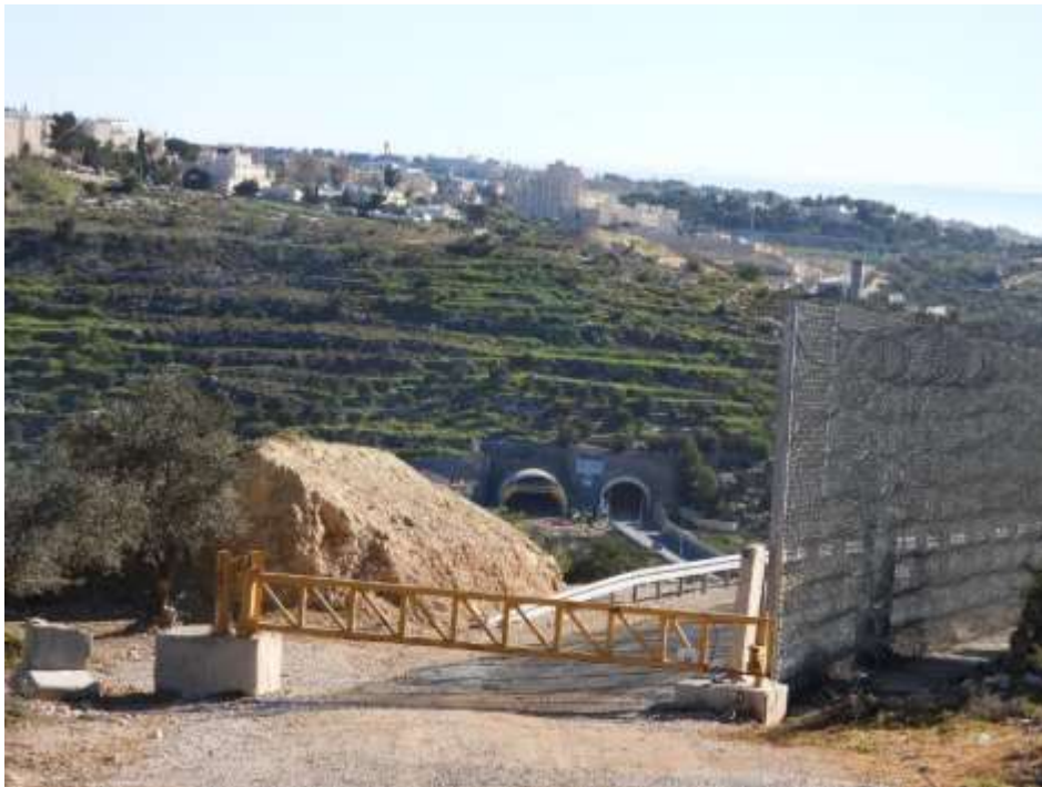
Fig. 33. Gate and part of the segregation wall installed by the occupation. Cremisan valley is to the left of the “Tunnel road” (settler road 60).
