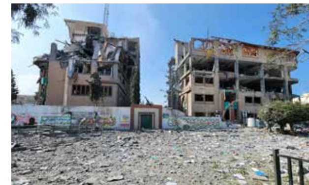
Fig. 1 Al-Azhar University main building during and after their destruction (Sources: Wafa Palestine News & Info Agency (top) and The Palestinian Information Center (bottom)).
